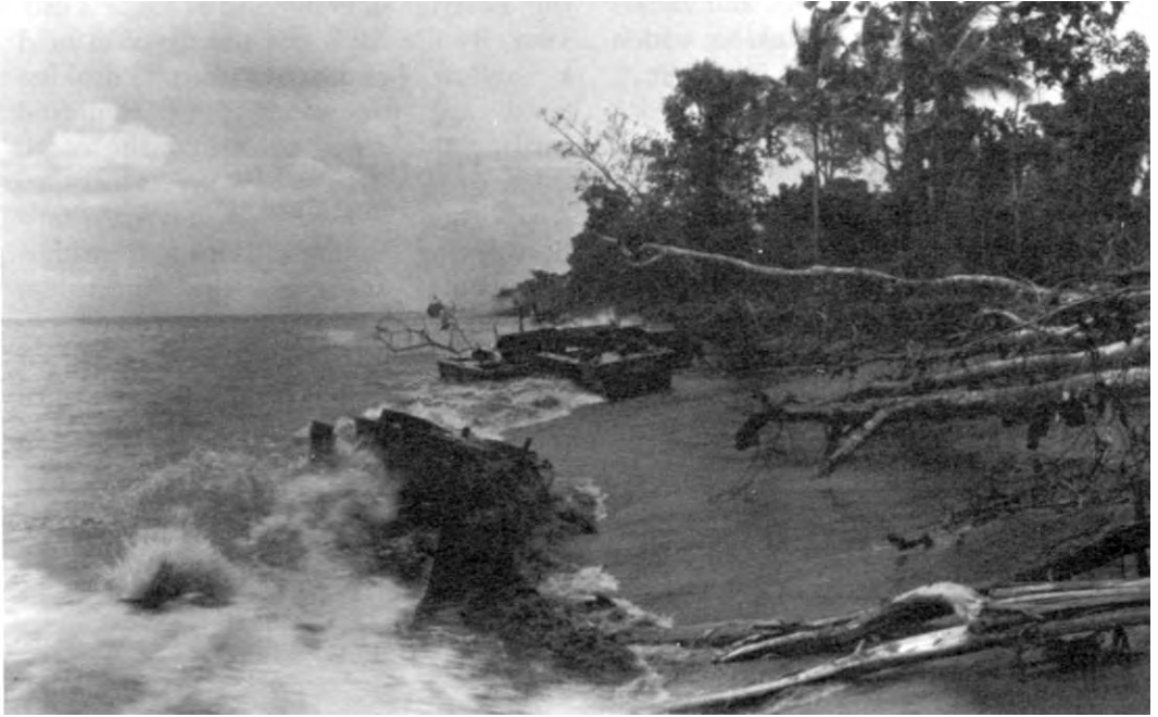
LCVP's ON THE BEACH AT EMPRESS AUGUSTA BAY damaged by the rough, driving surf.
