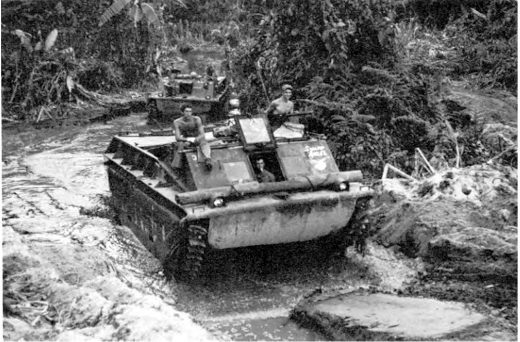
AMPHIBIAN TRACTORS LVT (1), carrying supplies and ammunition, move inland over a muddy trail.
