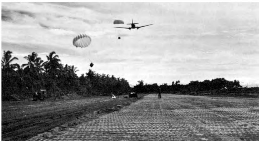
C-47 AIR-DROPPING SUPPLIES on a partially completed airstrip.
